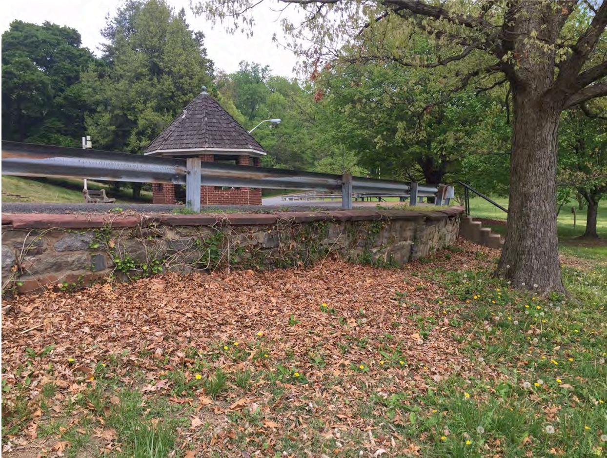
**Figure 5: Existing Conditions of Retaining Wall in proposed location of intersection with the new water line.**
