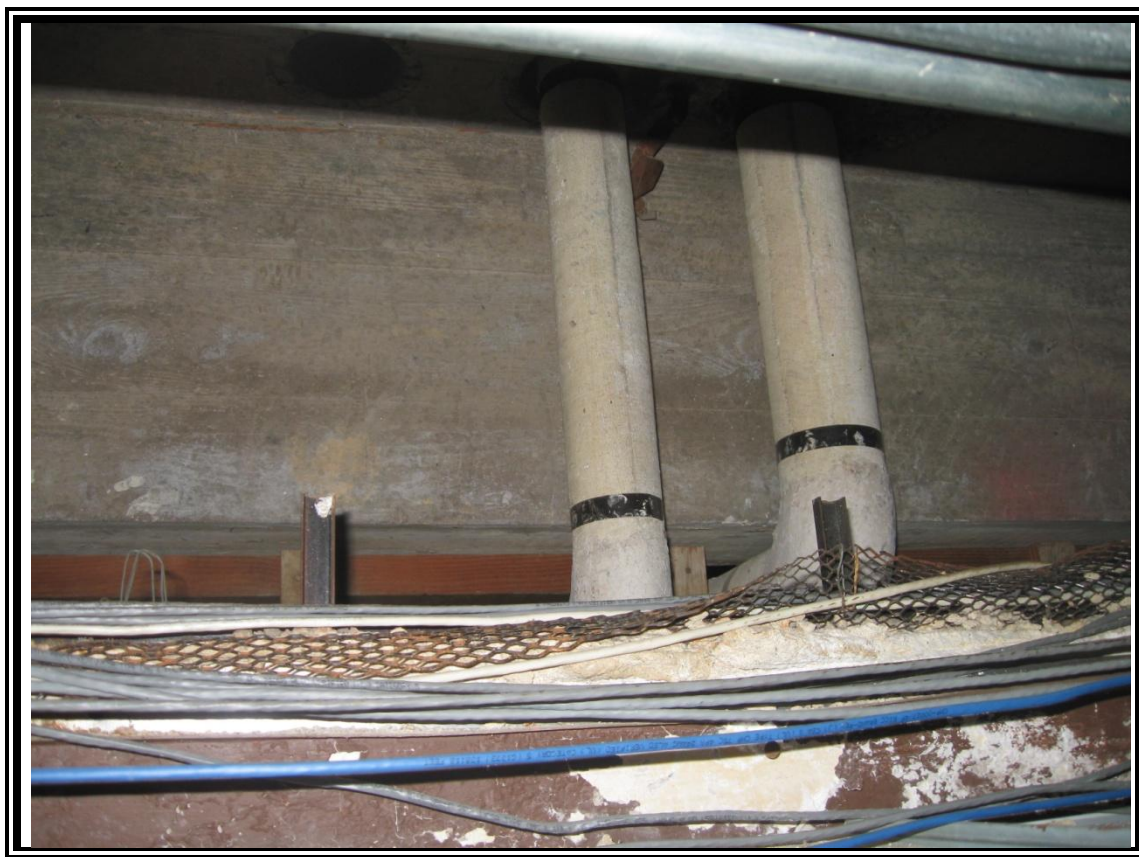
11. View of asbestos-containing air-cell and mudded pipe fitting insulation.
