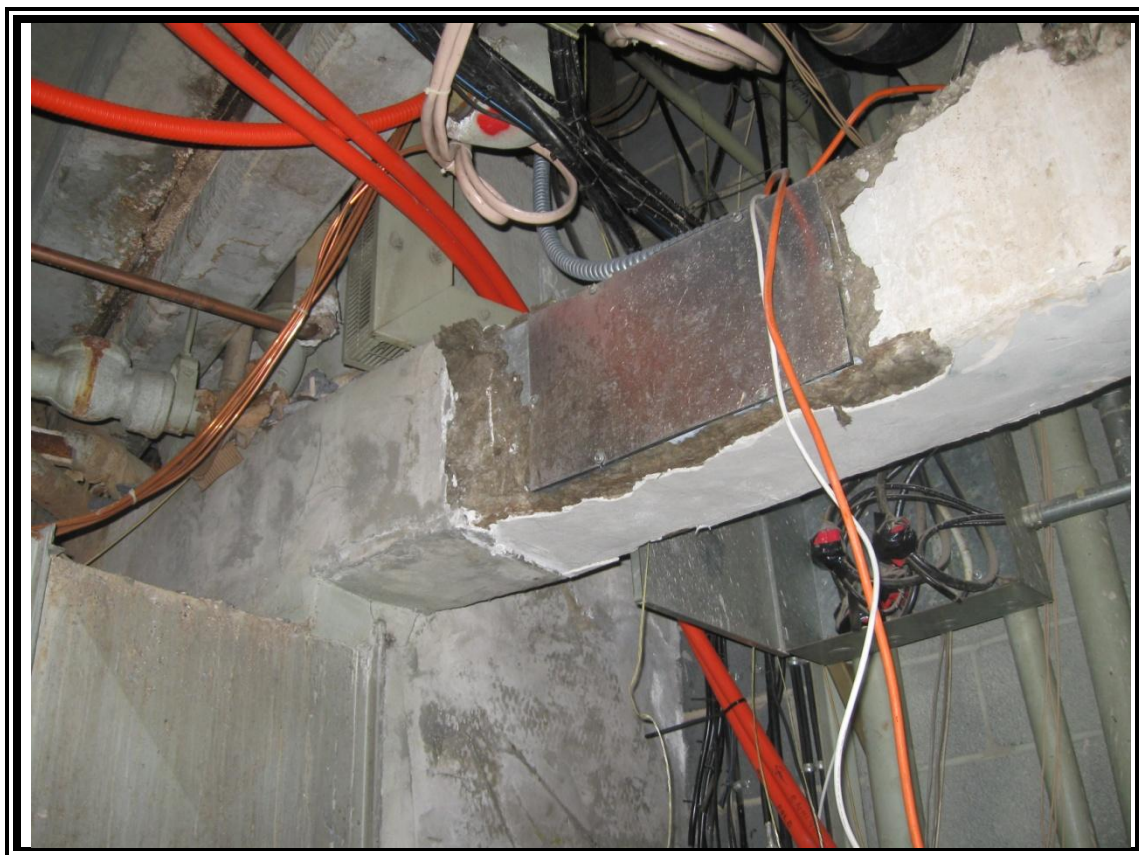
8. View of asbestos-containing HVAC duct insulation.
