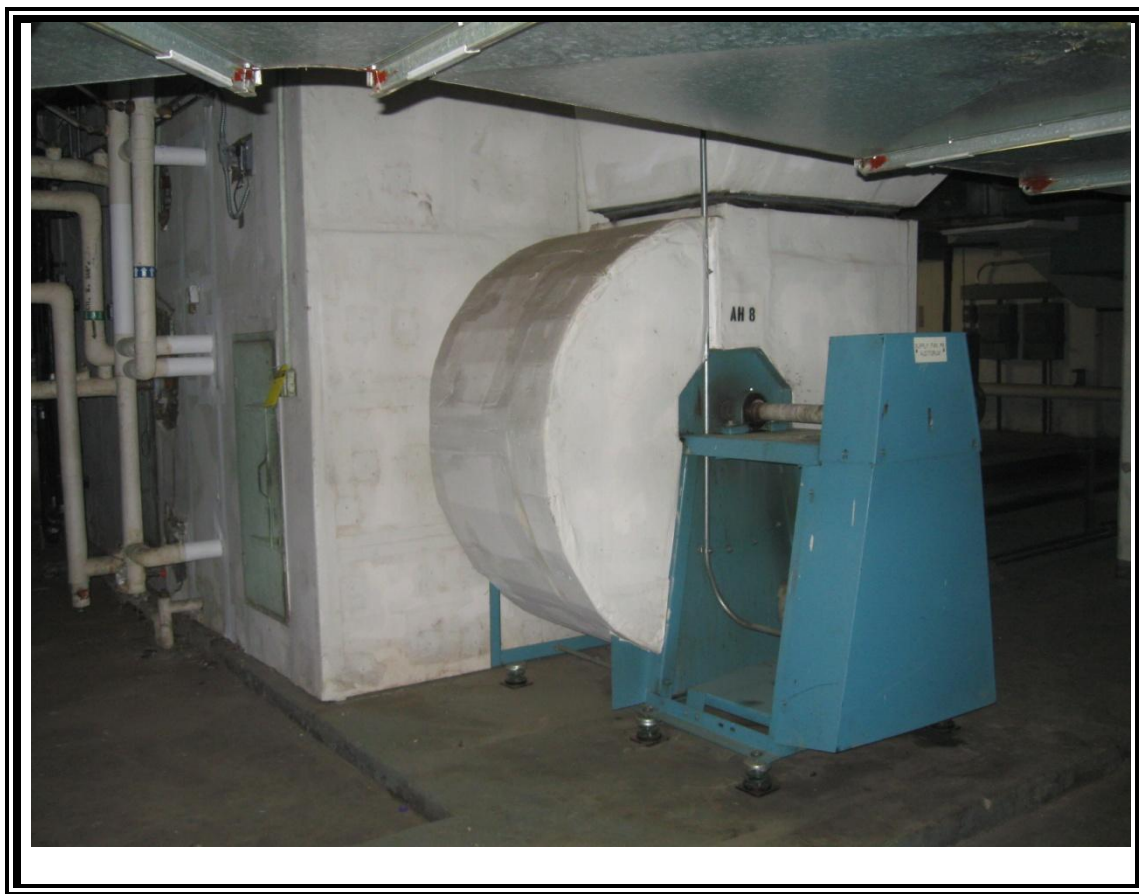
5. View of asbestos-containing Air Handling Unit #8 insulation.
