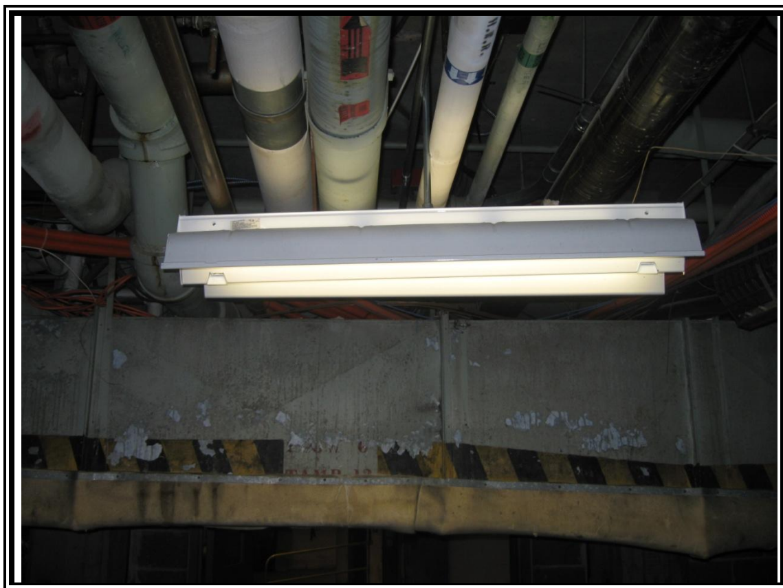
14. View of mercury-containing fluorescent lamps with PCB-containing ballasts.
