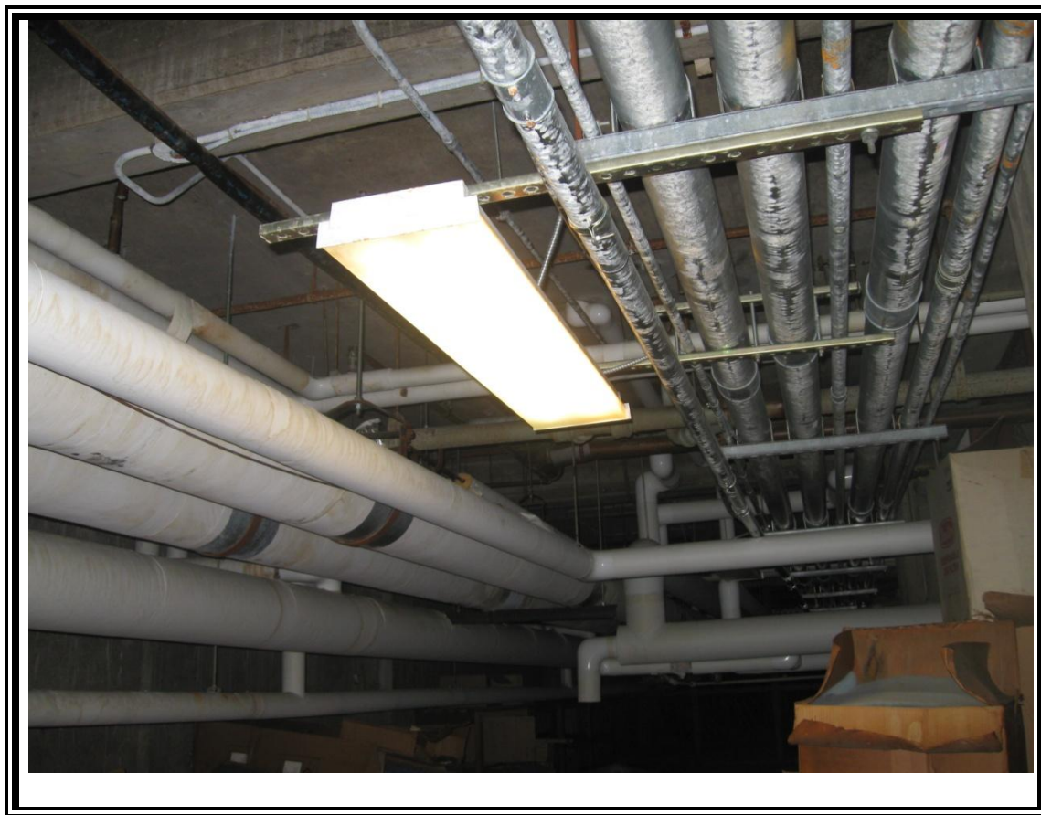
15. View of mercury-containing fluorescent lamps with PCB-containing ballasts.
