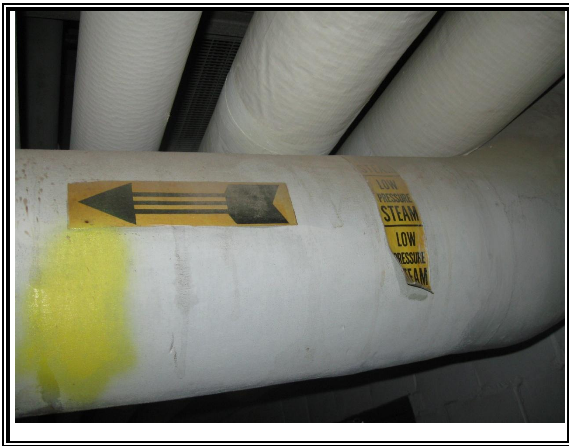
1. View of asbestos-containing steam pipe insulation.
