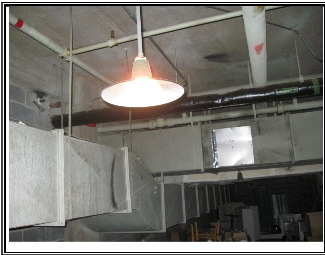
13. View of mercury-containing High Intensity Discharge (HID) lamps.
