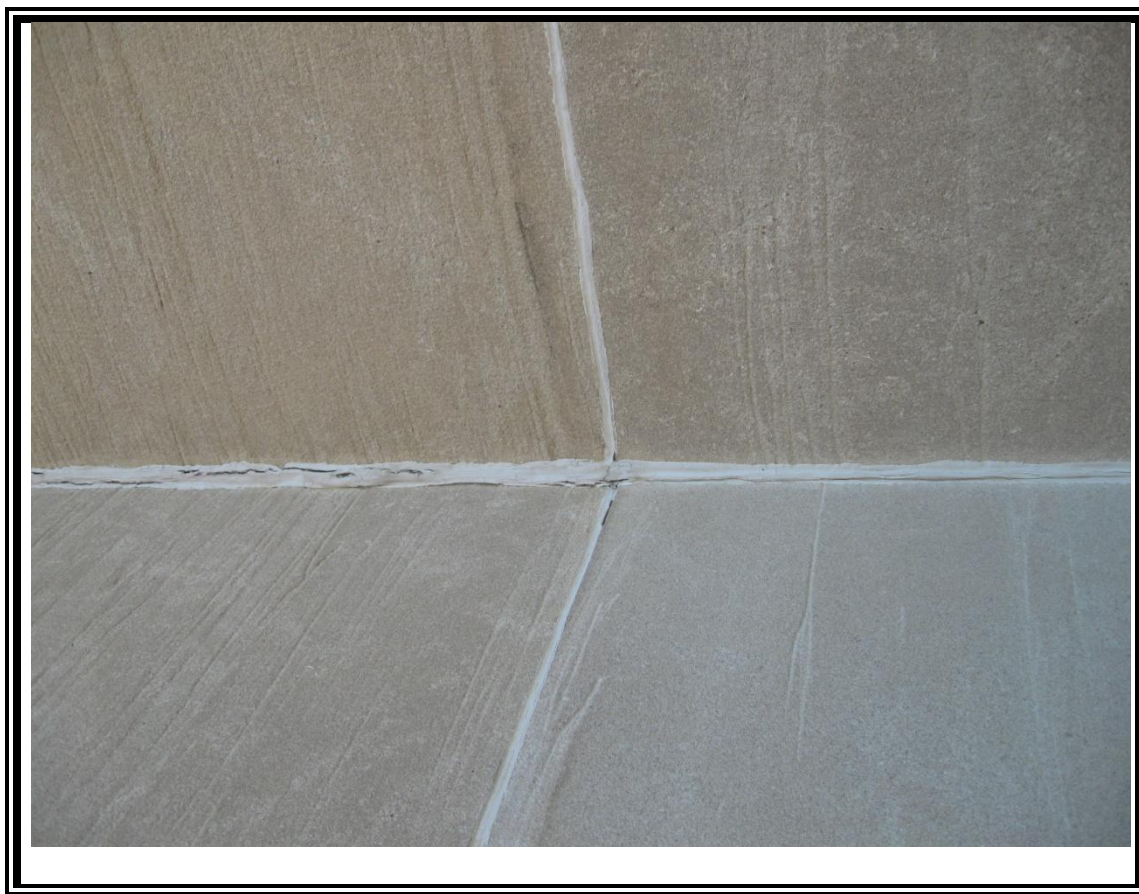
7. View of asbestos-containing exterior wall caulk.
