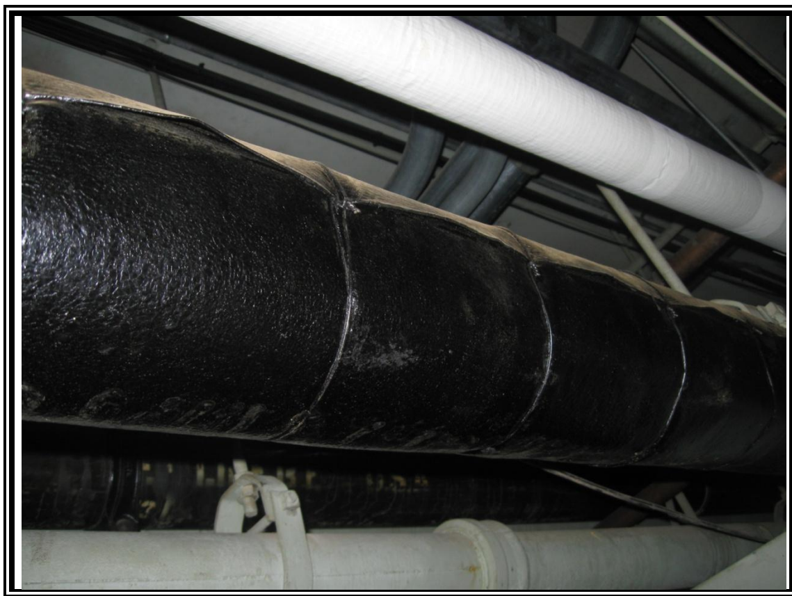
9. View of asbestos-containing black pipe wrap.
