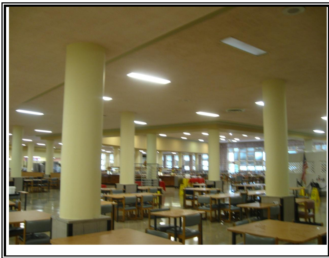
10. View of presumed asbestos-containing decorative ceiling plaster in the dining hall.
