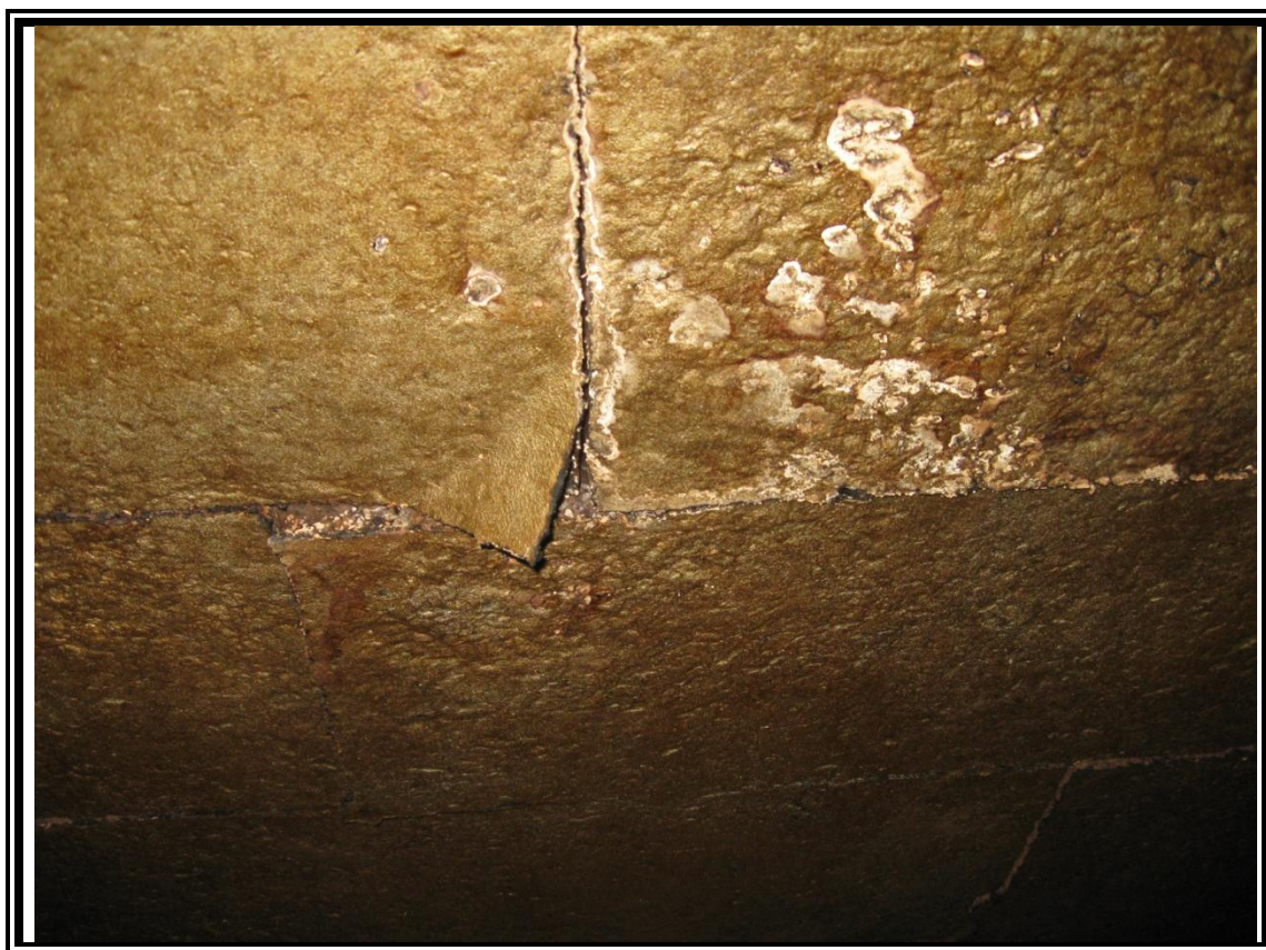
2. View of asbestos-containing paperboard ceiling.
