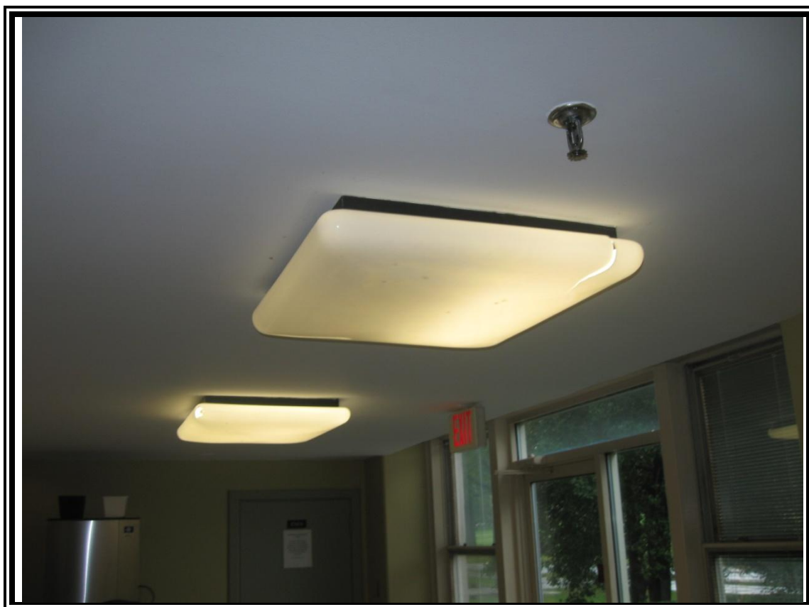
16. View of mercury-containing fluorescent lamps with PCB-containing ballasts.
