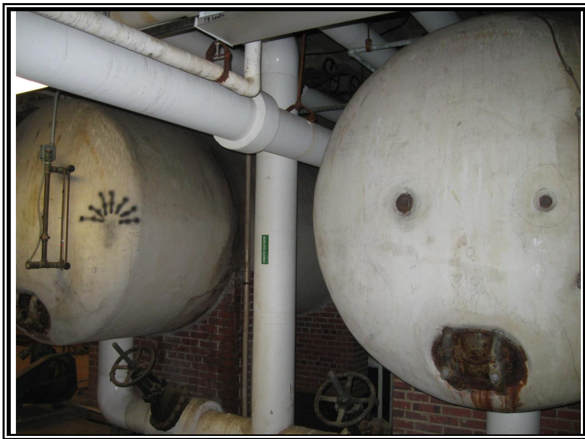
3. View of asbestos-containing hot water tank insulation.
