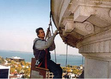
The use of special access methods may be necessary for close-up investigation of building elements. At the Wisconsin State Capitol, project architects and engineers used rappelling techniques. Photo: Wiss, Janney, Elstner Associates, Inc.
