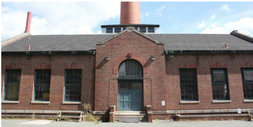
AFRH-Washington, DC Power Plant 2013
