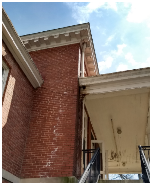
FIGURE 44: STORM DRAIN NOT SHEDDING WATER EFFECTIVELY AT HOSTESS HOUSE
