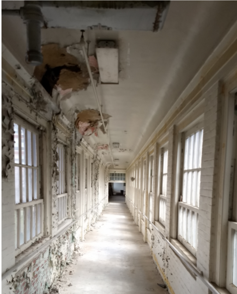
FIGURE 54: MESS HALL CORRIDOR SHOWING SIGNS OF WATER INFILTRATION AND ROOF DAMAGE
