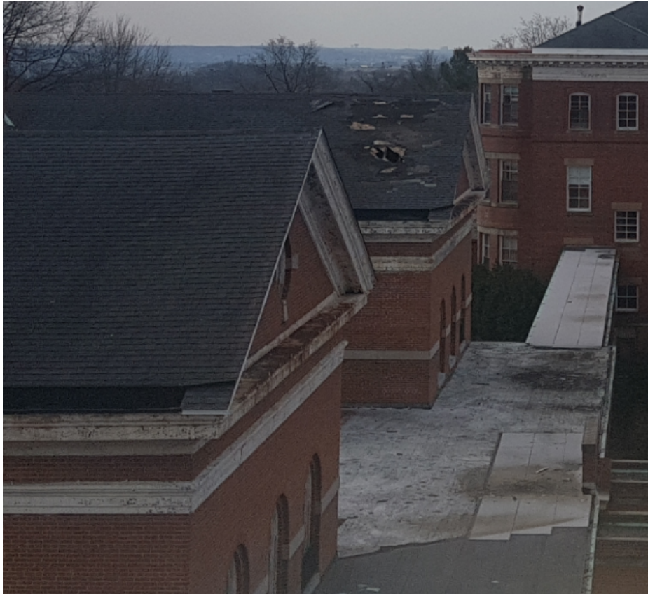
FIGURE 49: HOLE IN MESS HALL ROOF AND DAMAGED ROOFING AT MESS HALL CORRIDOR
