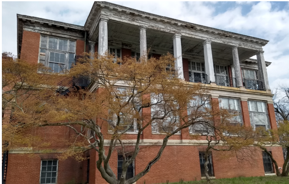
FIGURE 39: DETERIORATED SOFFIT & GOOD CONDITION BRICK WALLS AT BARNES
