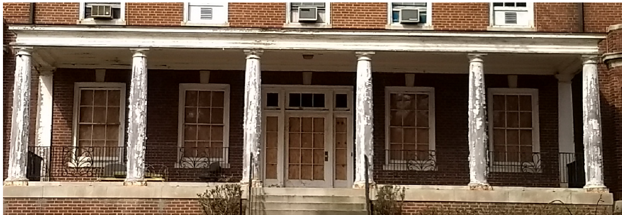
FIGURE 45: WOODEN EXTERIOR PORCH SOFFIT SHOWING SIGNS OF WEATHERING AND DETERIORATION
