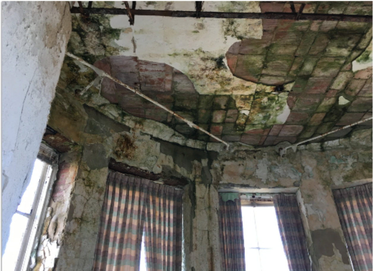
FIGURE 41: WATER DAMAGE AT THE FORWOOD SOLARIUM CEILING
