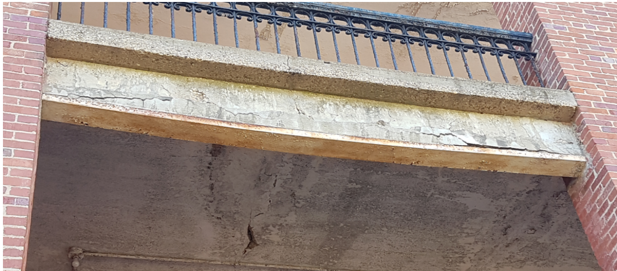
FIGURE 37: EXTERIOR STEEL BEAM WARPING AND CONCRETE SPALLING AT BARNES 2 ND FLOOR EAST SIDE
