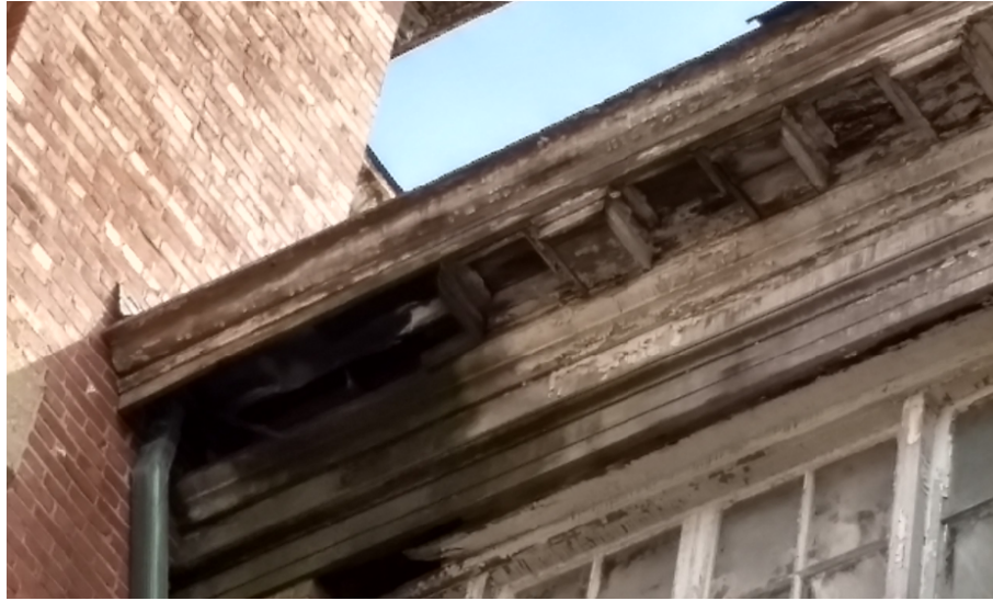
FIGURE 38: DETERIORATED SOFFIT AT BARNES
