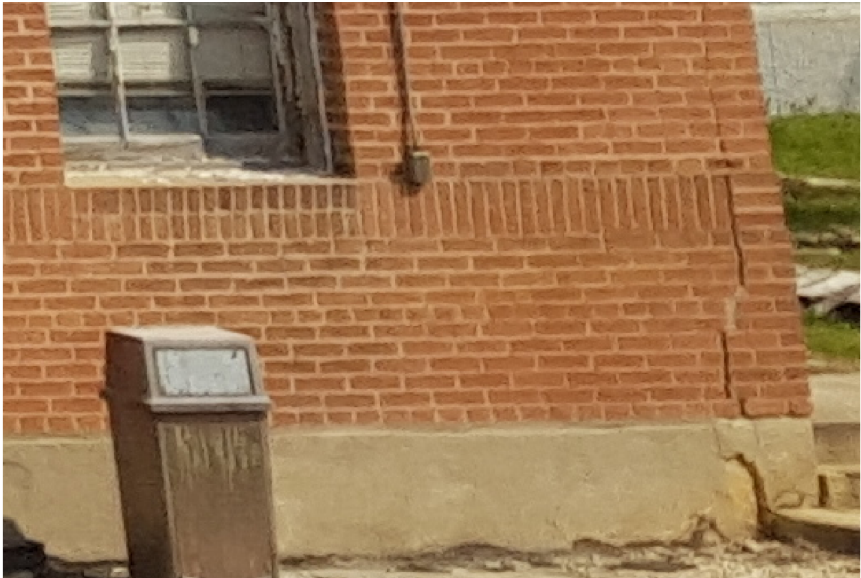
FIGURE 53: VERTICAL CRACK CAUSED BY SHRINKAGE AT MESS HALL SOUTH EAST CORNER
