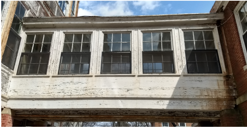
FIGURE 43: HOSTESS HOUSE WALKWAY TO FORWOOD SHOWING WOOD DETERIORATION
