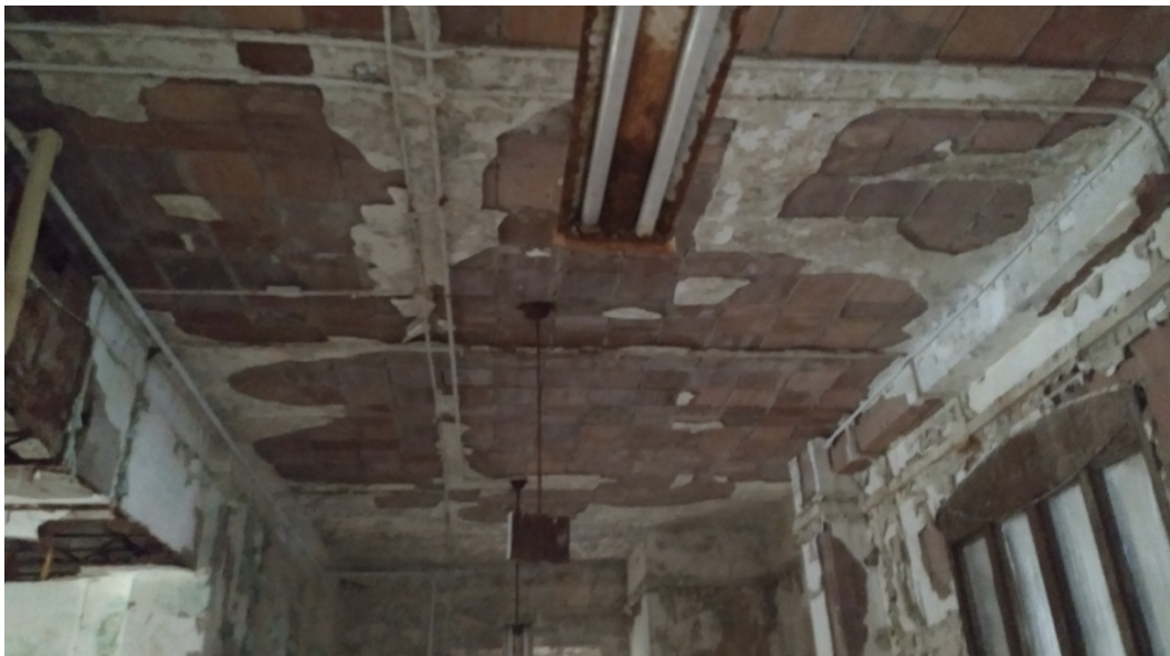
FIGURE 17: STRUCTURAL TILE FLOOR
