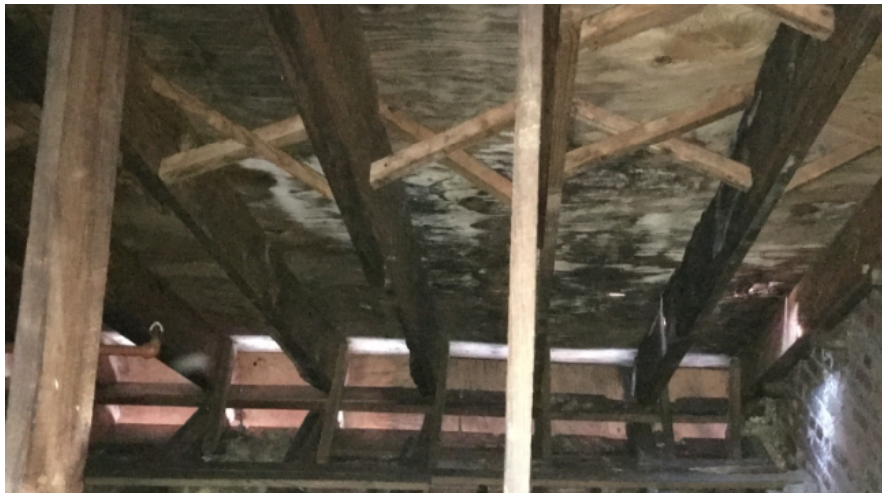
FIGURE 48: ROTTING WOOD SHEATHING, MISSING SHINGLES, AND ROTTING WOOD BEAMS AT MESS HALL ROOF
