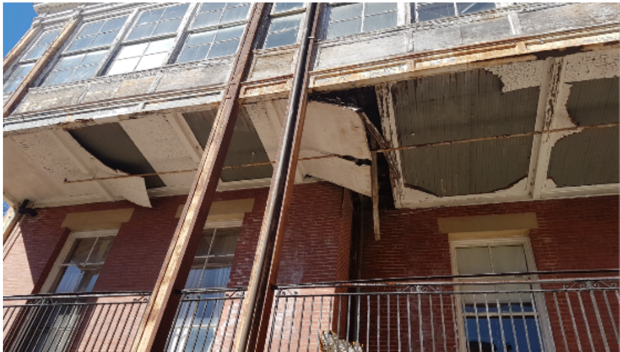
FIGURE 40: DETERIORATED SUN ROOM SOUTH SIDE OF FORWOOD
