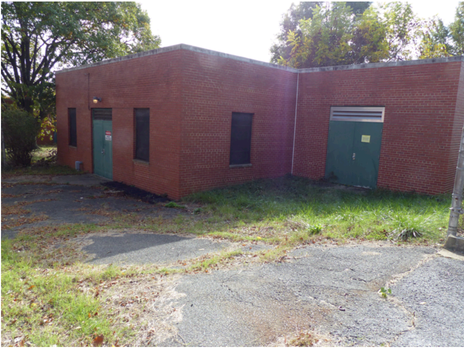
Image 6: Building 71 – Main Substation (Non-Contributing)
