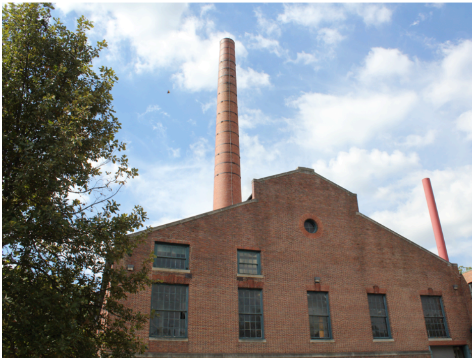
Image 3: Building 46 – Heating Plant (Contributing, Supporting)
