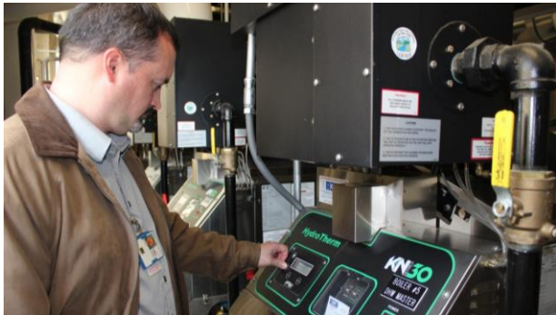
Facilities Manager Justin Seffens monitors energy use in the Boiler Room.
