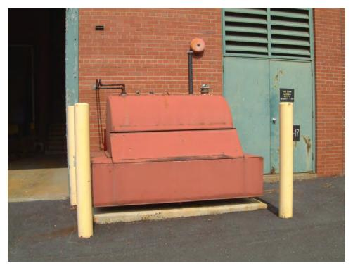
Photo 5: Above ground diesel storage tank for Building 74 emergency generator.
