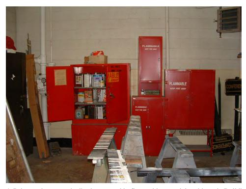
Photo 4: Paints, solvents, and adhesives stored in flammable materials cabinets in Building 73.
