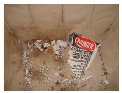
Photo 11: Asbestos debris in hamper in former laundry facility of Building 46.
