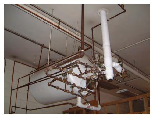
Photo 10: Asbestos insulation on piping and hot water tank in Building 77.
