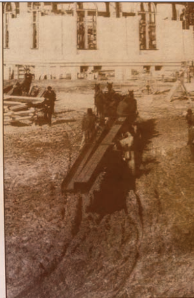
Above: By November 1908, most of the structure was complete. Manual cranes on each corner were operated by "pony engines" at the bottom to carry stone and supplies to the roof. Right: Horses pull steel beams to the construction site.
