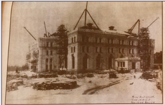
Above: By November 1908, most of the structure was complete. Manual cranes on each corner were operated by "pony engines" at the bottom to carry stone and supplies to the roof. Right: Horses pull steel beams to the construction site.
